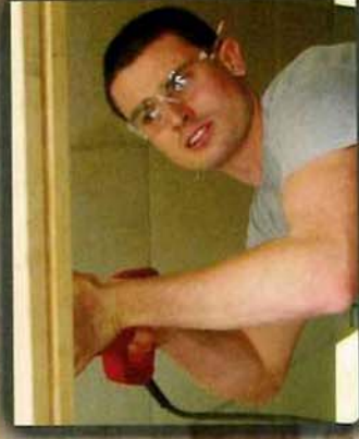
Jimmy Campbell using the Sawzall to cut off the unwanted nails
